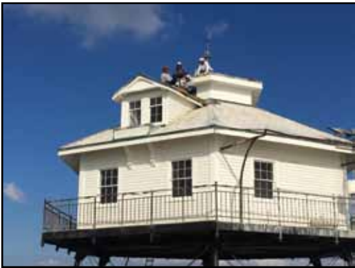
Workers help to repair Middle Bay Provided by Stephen Quinlivan
